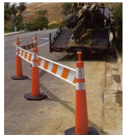
Direct traffic with 42" cones and optional plastic barricade panels
